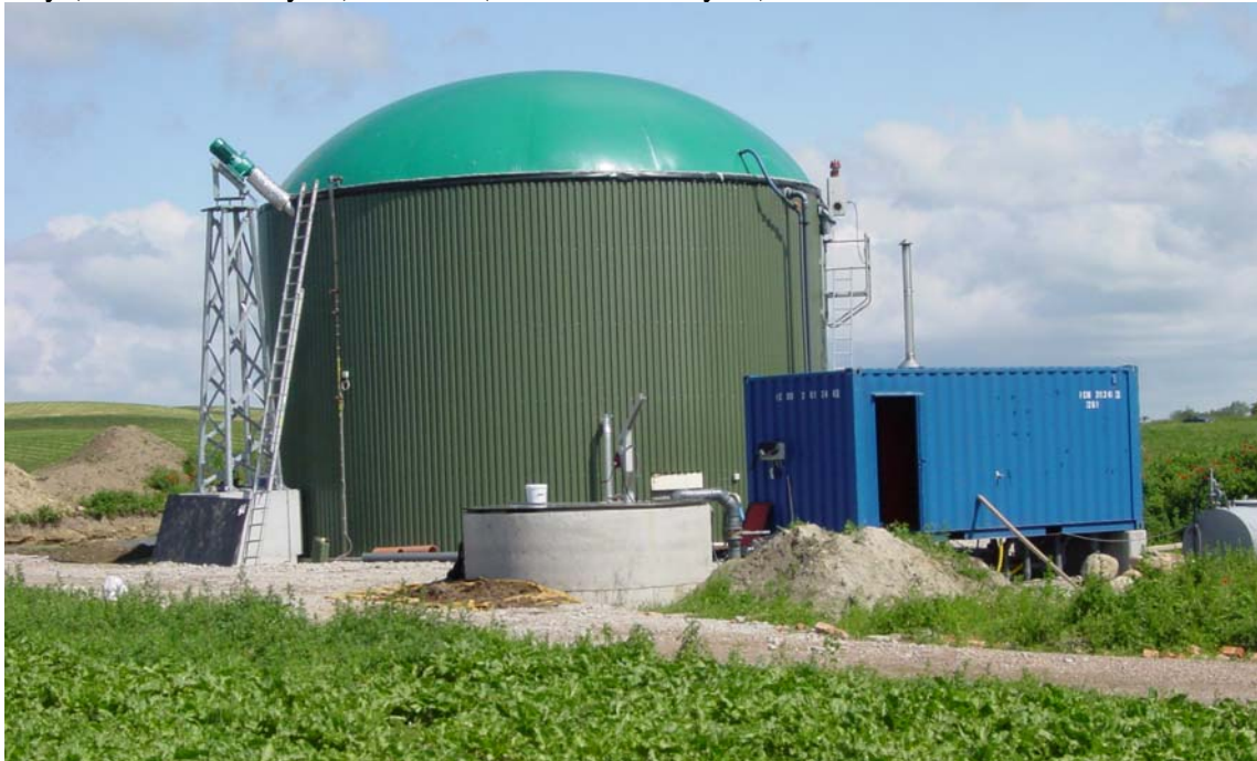
Figur 1: Hagavik biogas plant
