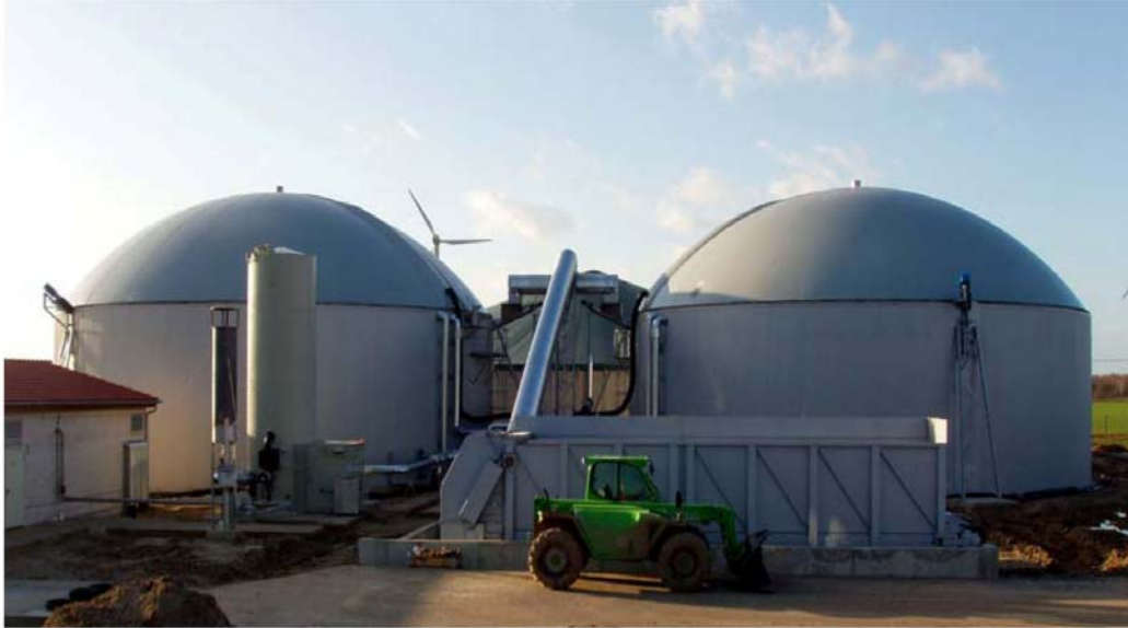
Figur 8: Hohenberg-Krusemark biogas plant
